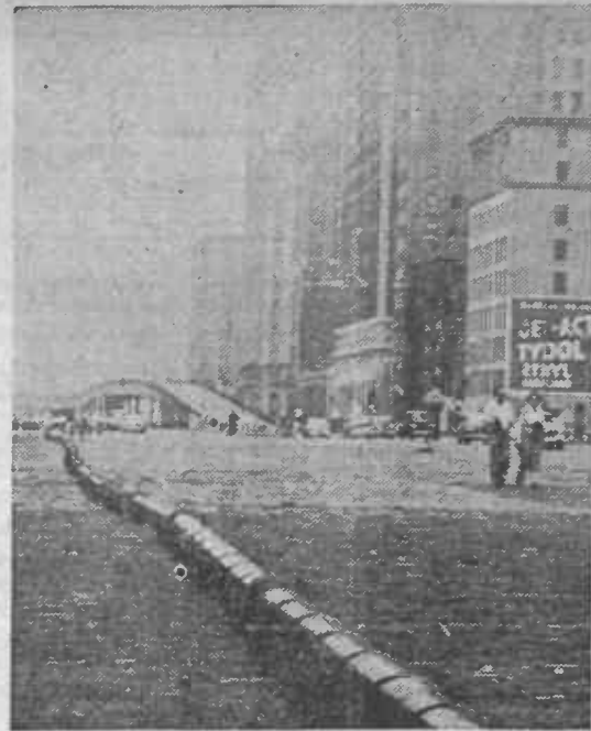
DEMONSTRATION OF PIPE in New York City which can be laid quickly over rough terrain to carry water for fire fighting, city water supply or to pump out flooded areas. This flexible-
